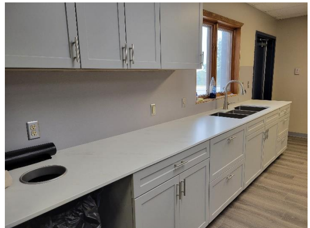
CLS Kitchen Remodel
